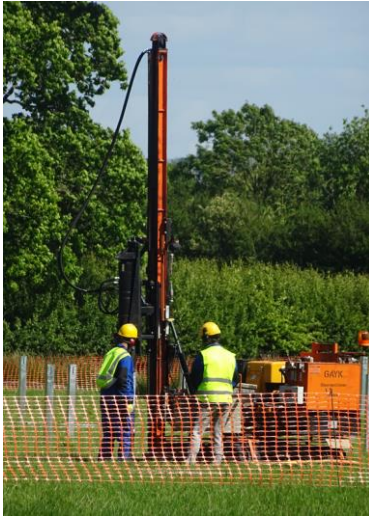
Photos 18 and 19: Example of Leg Piling and Panel Moving Equipment
