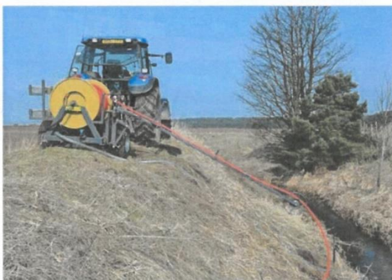
Figure 23. Drain jetting
