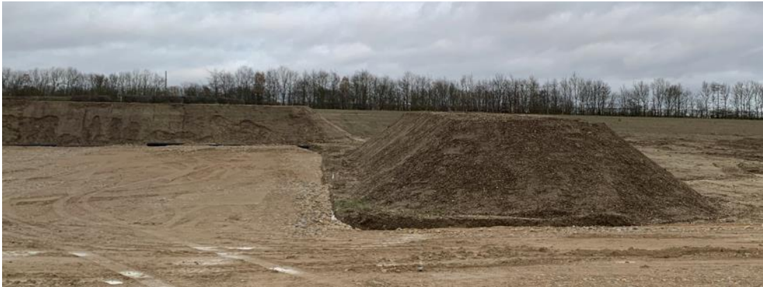
Photo 12: Topsoil Storage Bund
