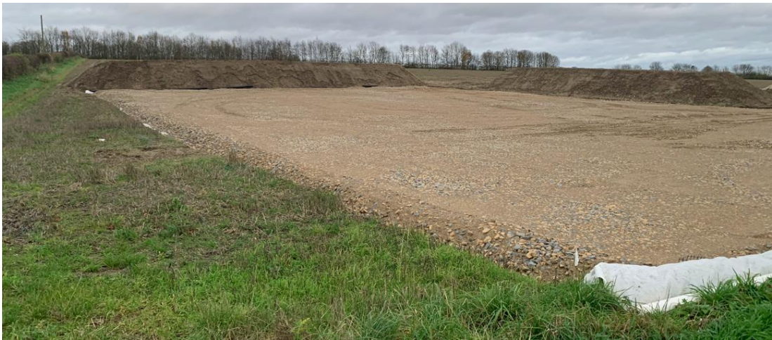
Photo 10: Newly-laid Construction Compound (Elsham-Lincoln Pipeline)
