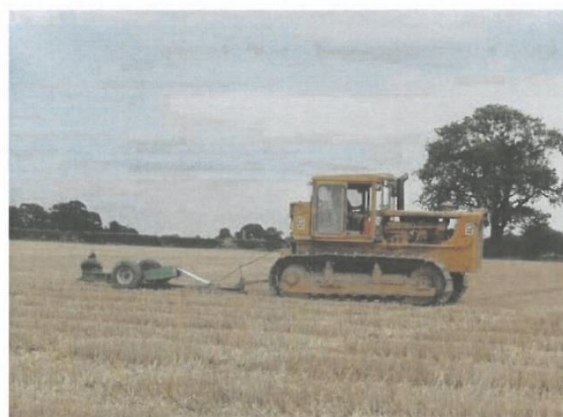
Figure 30. Installing mole drains
