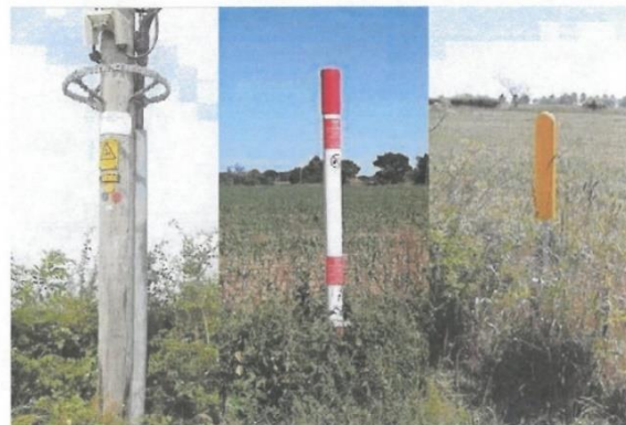
Figure 18. Signs indicating potential underground hazards
