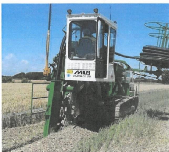
Figure 31. Installing land drains with laser gradient control
