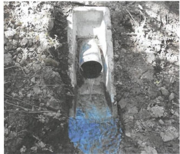
Figure 38. Precast concrete headwall (type K)
