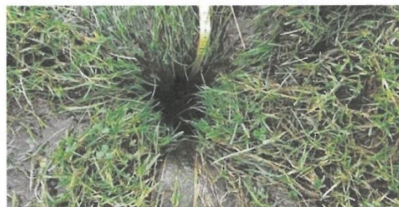
Figure 17. A 'blow hole'
