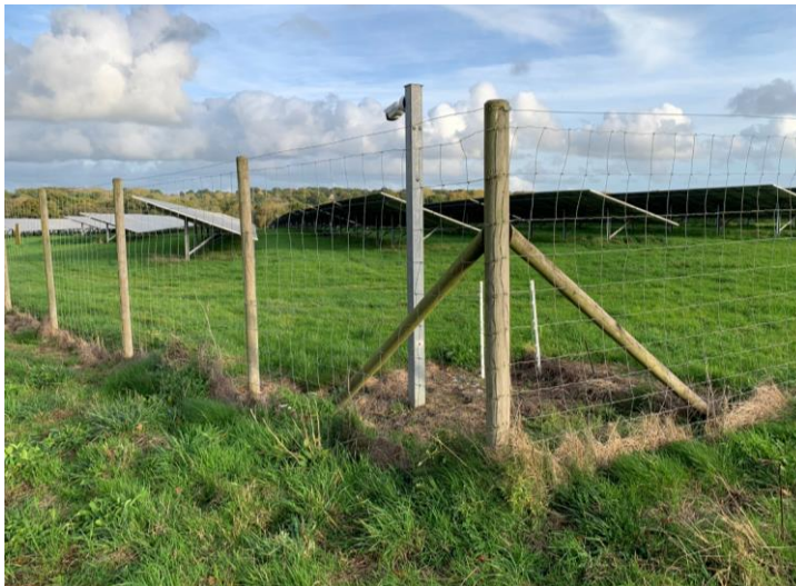
Photos 26 and 27: CCTV Poles and Fencing
