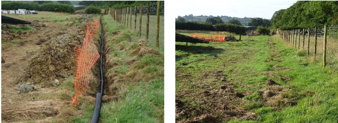
Photos 22 and 23: Cable Installation
