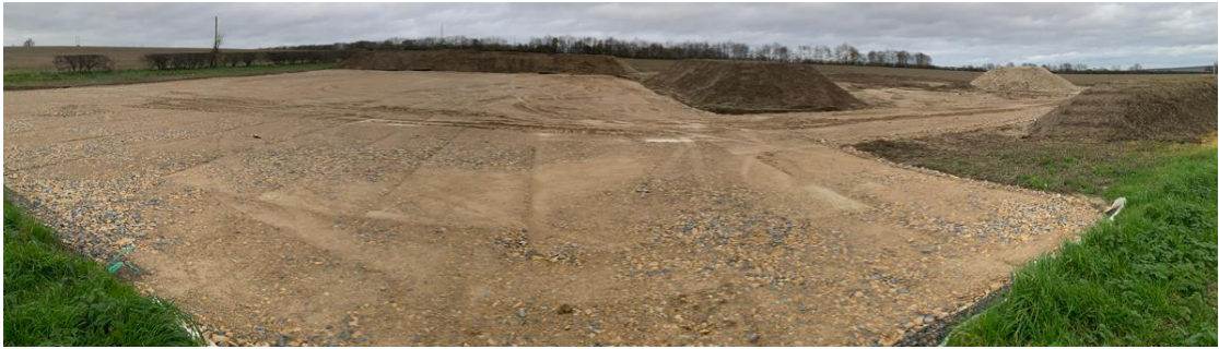
Photo 28: Example Base Construction
