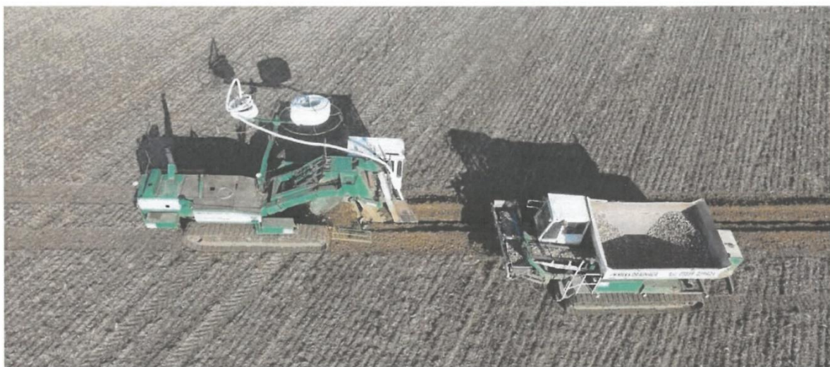
Figure 28. Installing land drains and stone backfill
