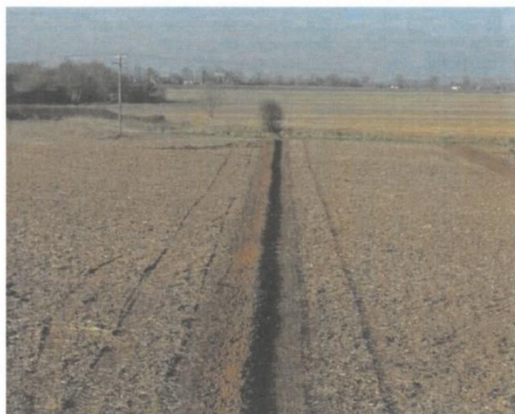
Figure 29. Recently installed drains
