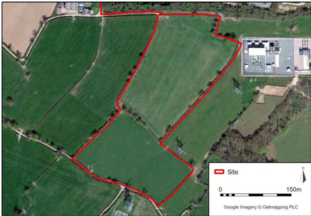
Figure 38: 2015 Google Satellite Imagery of the BESS Site © Getmapping PLC
