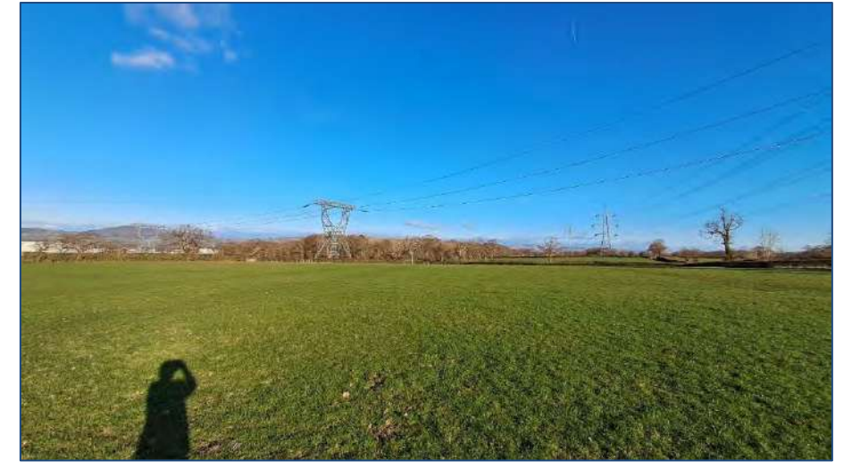
Photo 16: BESS Site, viewed from south-west looking south-east
