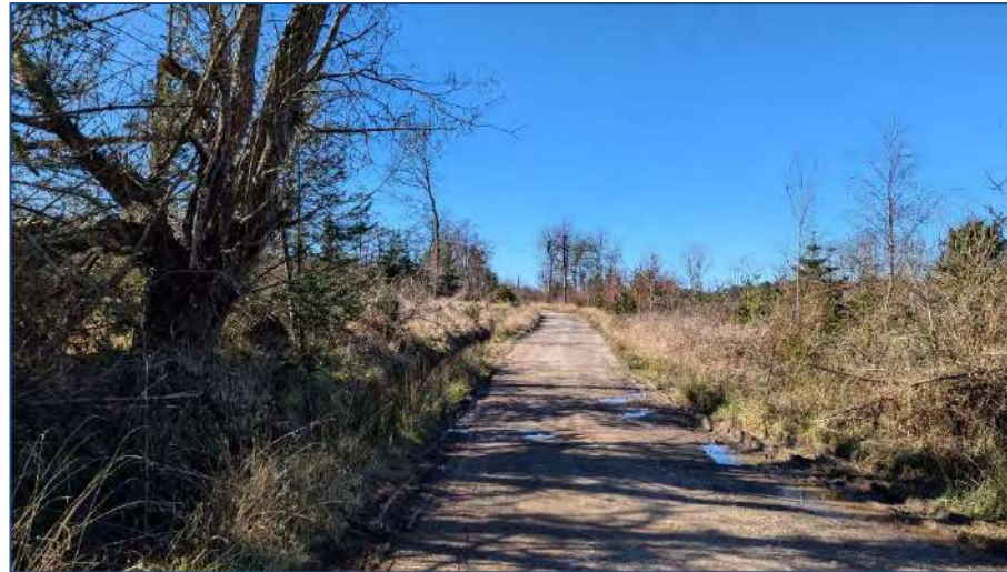
Photo 22: Cable Corridor, route in the north of Kinmel Park, looking west
