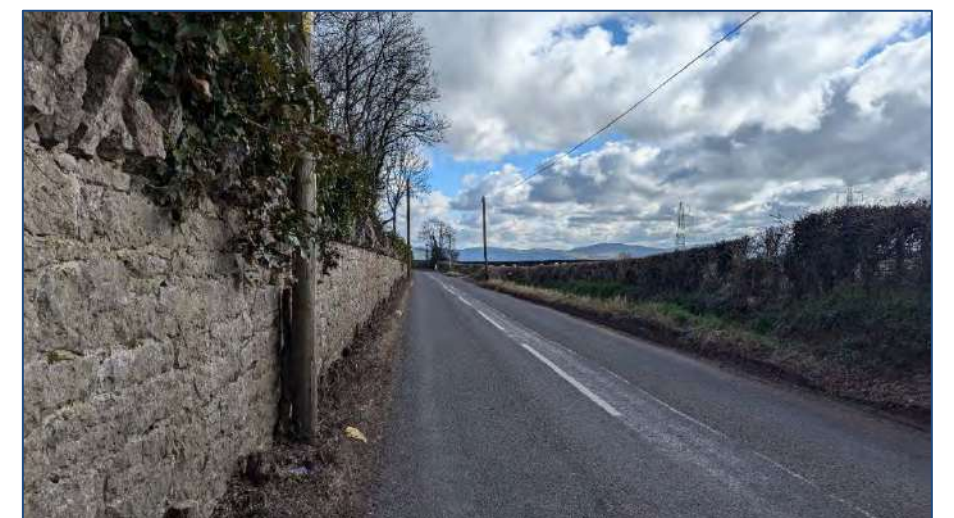
Photo 26: Cable Corridor, route along Roman Road, looking east
