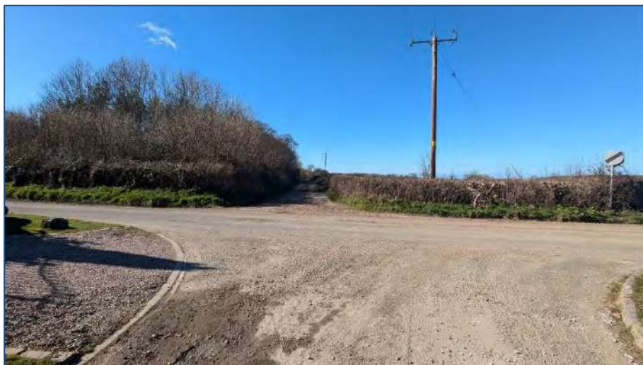
Photo 21: Cable Corridor, junction at the north-west entrance to Kinmel Park
