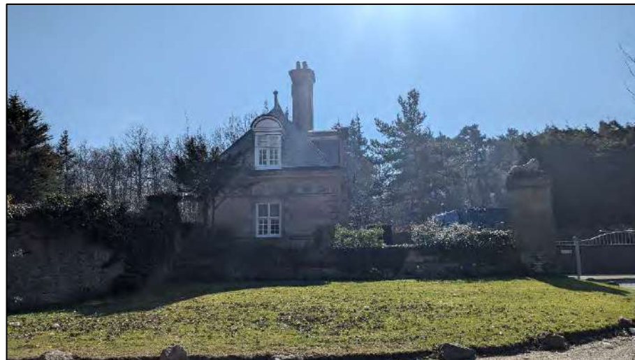
Photo 32: Llwyni Lodge and part of the Gate Piers
