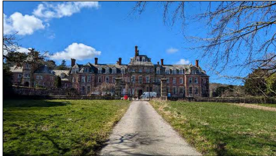
Photo 31: Kinnel Hall, front elevation and Entrance Screen to main entrance front
