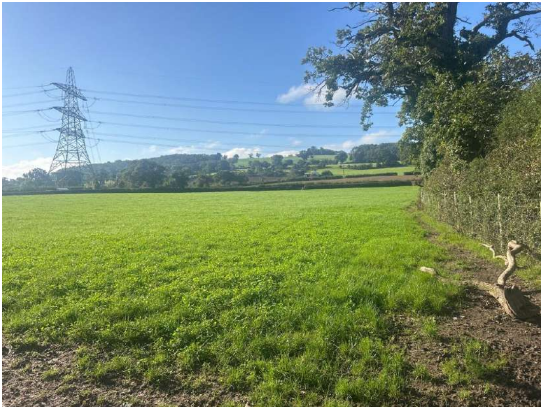
Plate 18: Field 29 BESS facing southeast from the northwest corner.
